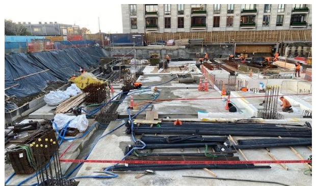
Zone 4 - Tanking and Ground Beam Reo
