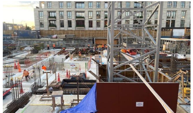
Zone 3 - Tanking and Slab Reo
