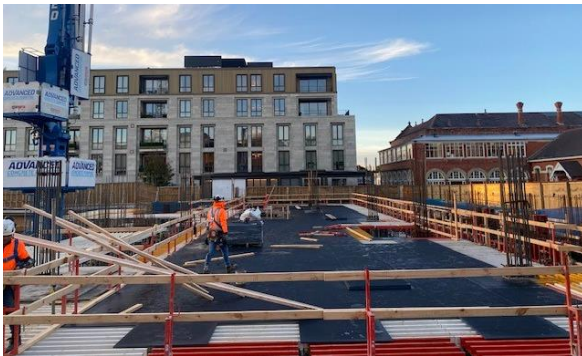
Area 1 - Gridflex install for Ground Floor
